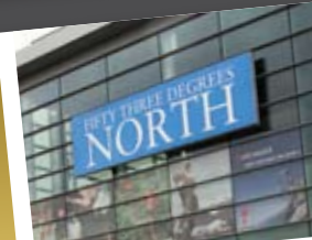
53 Degrees North Blanchardstown Retail Park, Dublin
